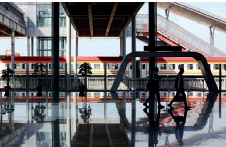
On October 16, a brand new train set off from the south station in Nairobi, traverses the picturesque mountains and grasslands to Naivasha. This marks the official opening of the first stage project of the Nairobi-Malabar standard railway undertaken by Chinese companies. Wang Teng
