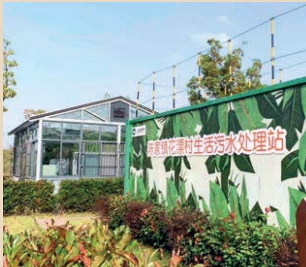
Sanitary sewage treatment station in Huapiao Village, East China's Zhejiang Province, October 29. Zhang Yuchai
