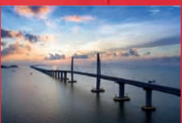
Hong Kong-Zhuhai-Macao bridge opens to traffic.
