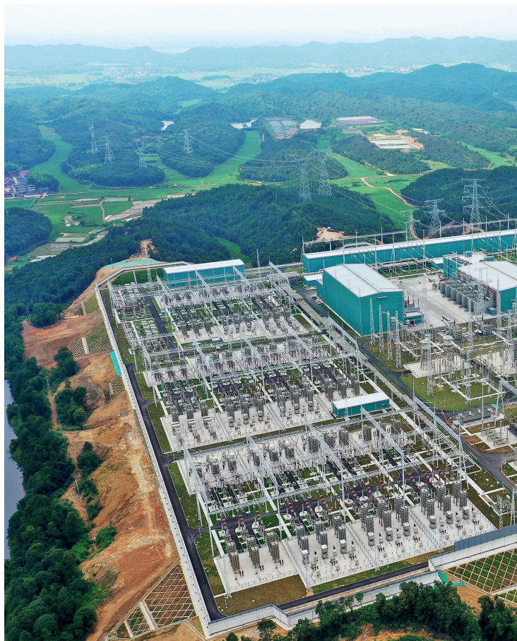
Aerial photo shows the Poyang Lake converter station in Fuzhou, Jiangxi Province, on June 18, 2021. The \pm 800\text{KV} UHVDC transmission project from Yazhong in Sichuan Province to Poyang Lake is officially put into operation on June 21, 2021, further expanding the power capacity to support regional green development. Xinhua
