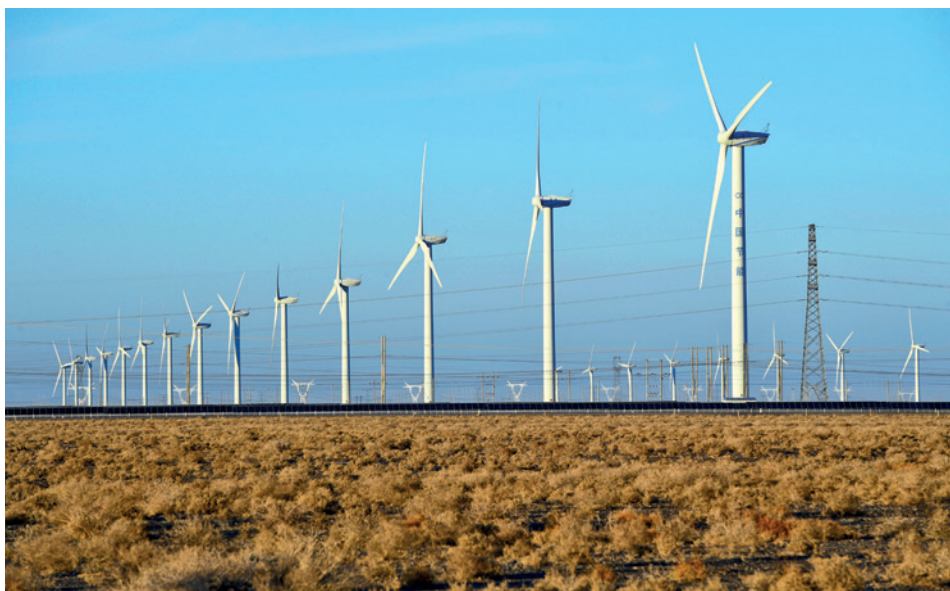
Photo taken on December 8, 2021 shows wind turbines at Changma wind farm in Yumen City of Gansu Province. Fan Peishen
